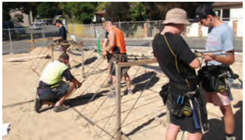
Making Reinforcing
